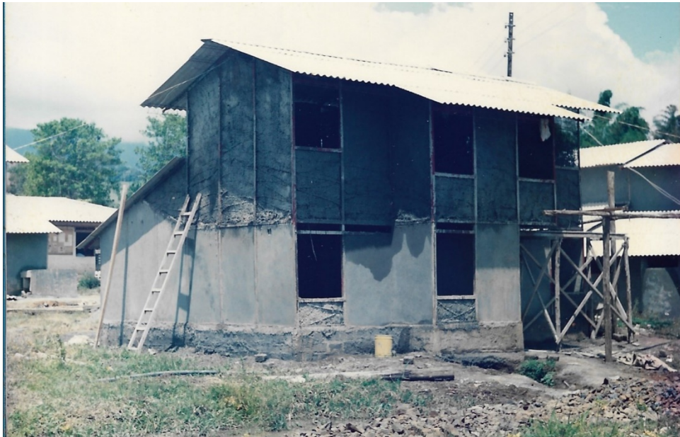
Figure 4 Construction of the tendon wall system
