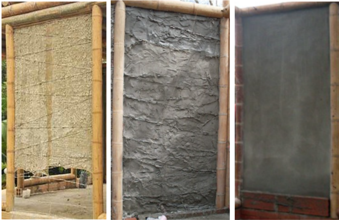
Figure 3 Construction of the tendon wall system
