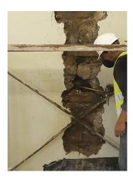
Peñaranda (2011) suggests that for a good rehabilitation against the appearance of cracks affecting the walls of a heritage building, "wooden keys" should be used. These are essential to reduce the seismic risk to which the affected masonry of the construction is subjected. The application of this system is intended to prevent the collapse of the building in the event of new natural phenomena (earthquakes or seismic movements).
