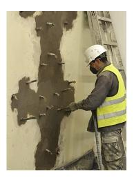
It should be noted that these injection mortars used for structural reinforcement were subjected to PUCE laboratory mechanical tests<sup>16</sup>, in order to measure their compressive strength. The values obtained allow the mechanical properties of the mortar tested to be assessed.
