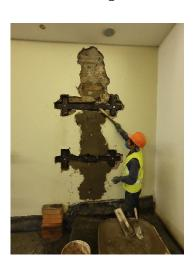
Once the stitching and unpicking was completed, the wooden keys were attached. Next, the plastering work was done to seal the masonry and then consolidate the wall with the mortar injection process.
