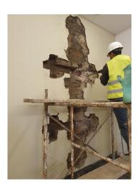
**Figure 17**Wooden key image protected with asphalt paint and wrapped with mesh. Anchoring with steel rod
