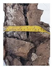
It should be noted that this process of verifying the presence of cracks by means of the shim method on the walls should be repeated on all the masonry to be subjected to a reinforcement process.
